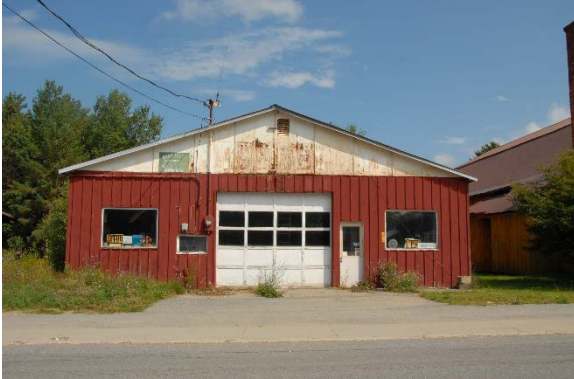
Townsend buildings existing condition
